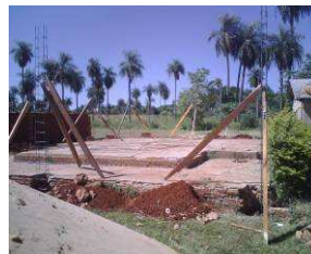
Photo taken after two days of work
