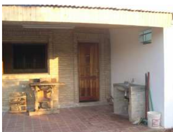
The new back porch.
