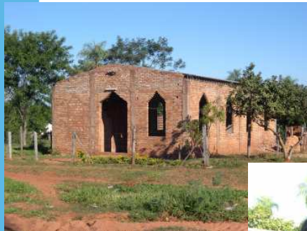
←Front of church looking from road.
